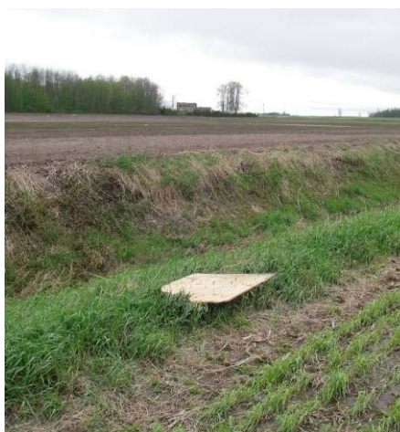
Photograph showing flight distance of a 4' x 4' sheet of plywood which originated from the house in the background. Of note is the trail of debris in the field and the nails still in the plywood.
